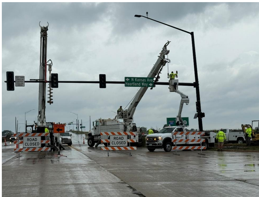
Removal and reinstallation of traffic signal pole at W Penn St / Heartland Way intersection
