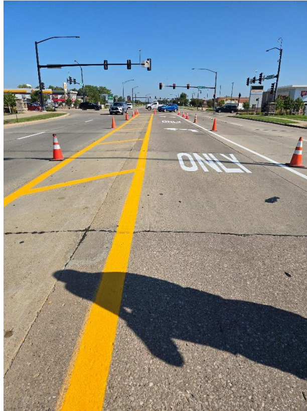
Painting operations on Ranshaw Way
